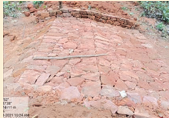
Loose Boulder Check Dam Hemgir, Sundargarh Mayurbhanj
