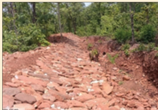
Graded Earthen Bund Banki Range, Sundargarh
