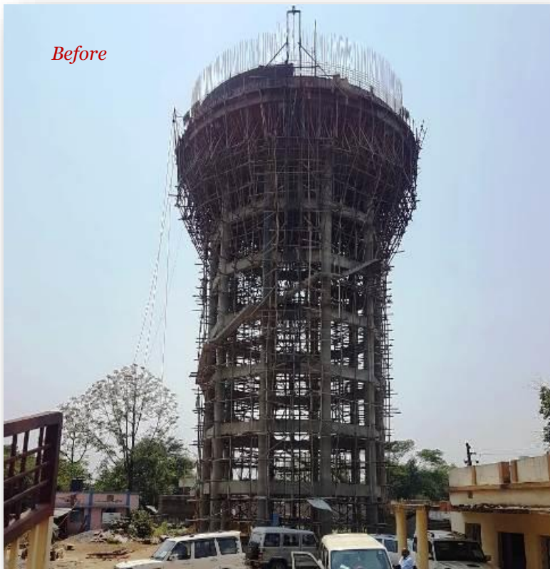
Construction of ESR at Rourkela Township area, under Rourkela PH division.
