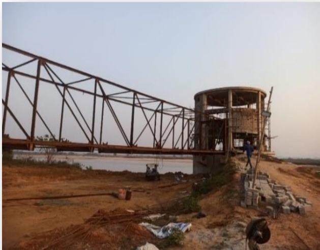
Under Construction Intake well at Sukinda block
