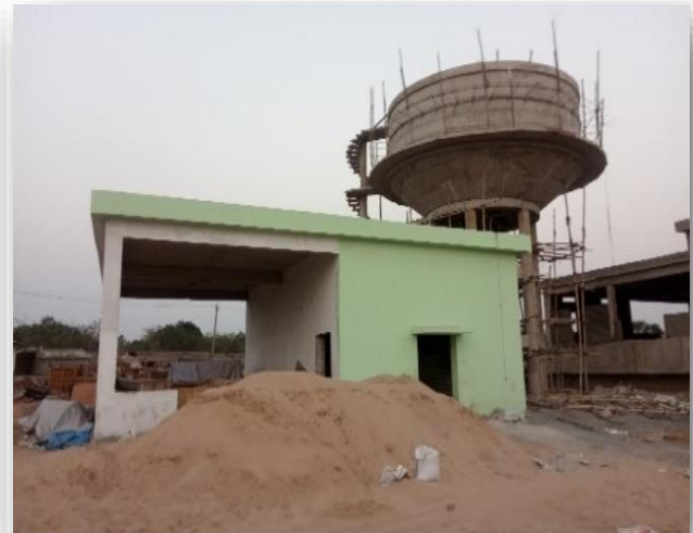
Under construction of WTP at Sukinda block
