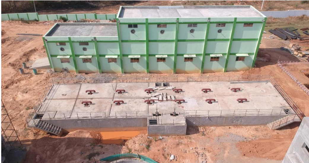
Under Construction WTP at Kusumi block, Mayurbhanj district
