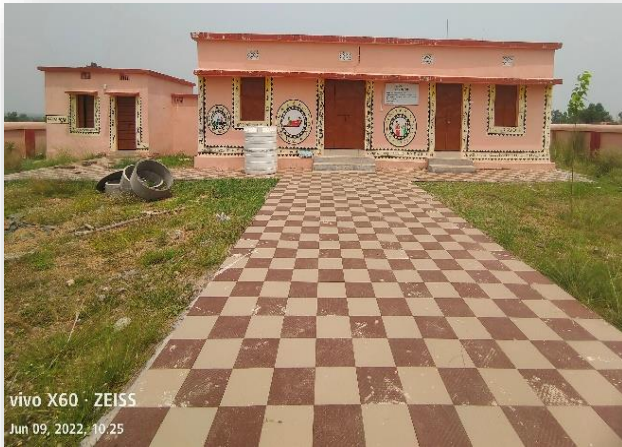
Newly constructed Basingi SC, Mayurbhanj
