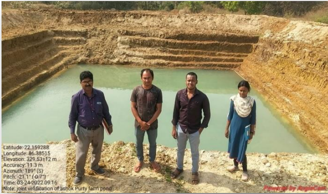
Construction of Farmpond to improving food security & nutrition
