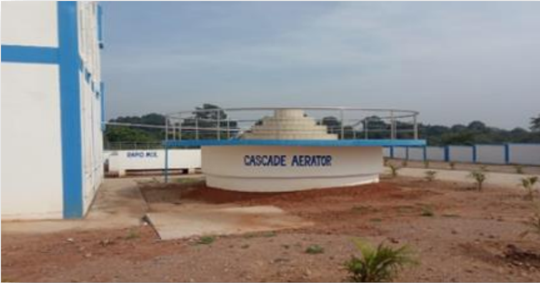
Cascade Aerator @ Keonjhar ULB
