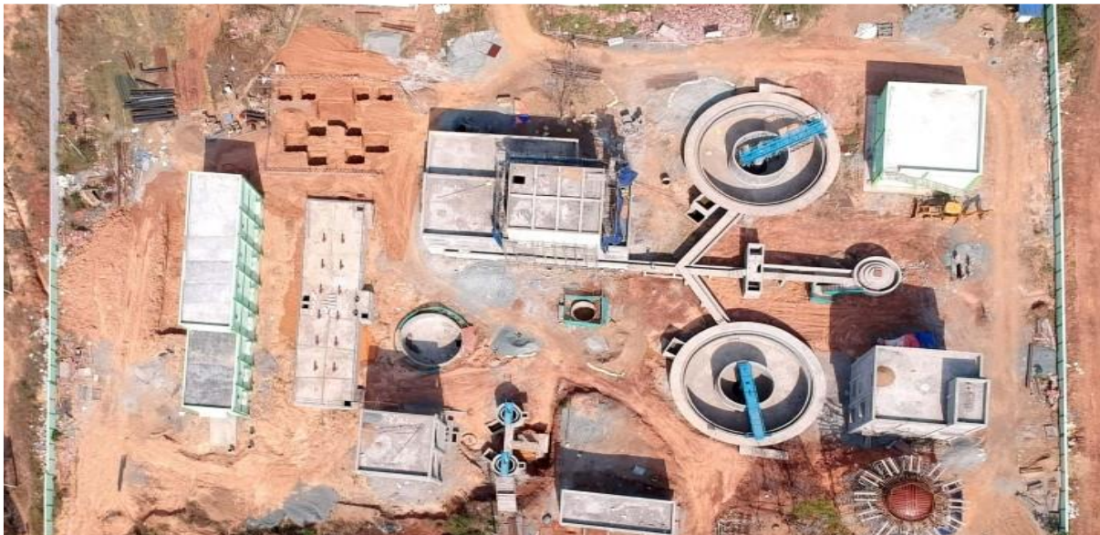
Under construction WTP at Rairangpur block, Mayurbhanj
