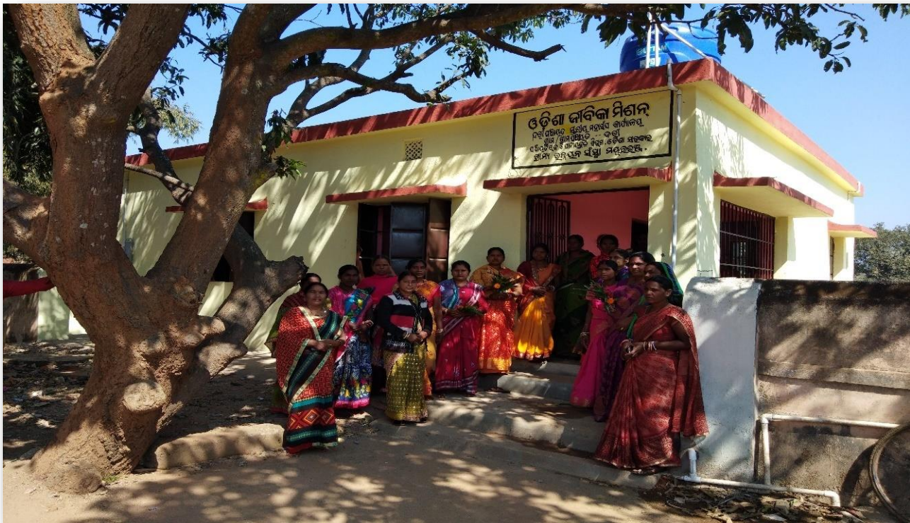
Newly constructed GPLF Building at Karanjia, Mayurbhanj
