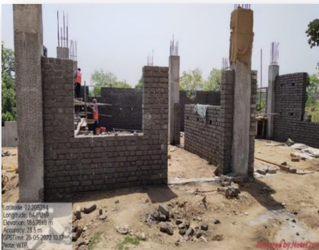
Construction of Admin building of WTP at Mega PWS
