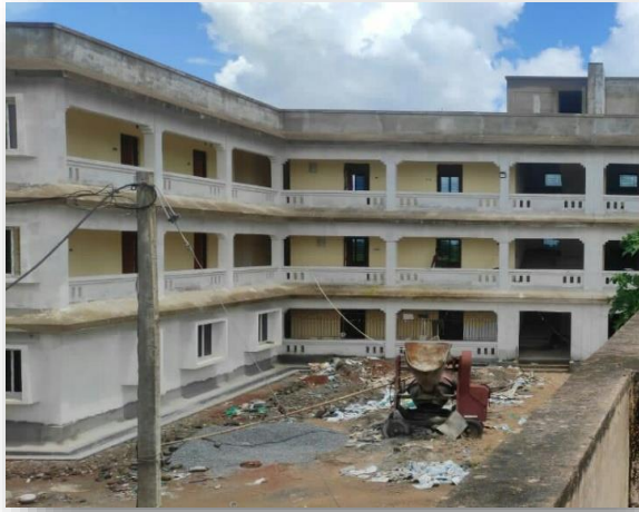
Girls Hostel, Baripada, Mayurbhanj
