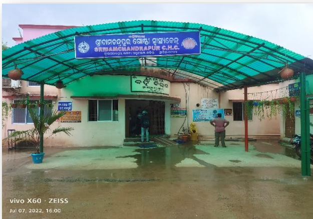
Sri Damdamchandrapur CHC renovation
