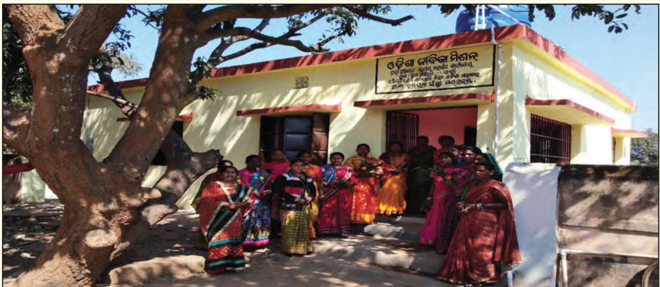
Newly constructed GPLF Building at Karanjia, Mayurbhanj
