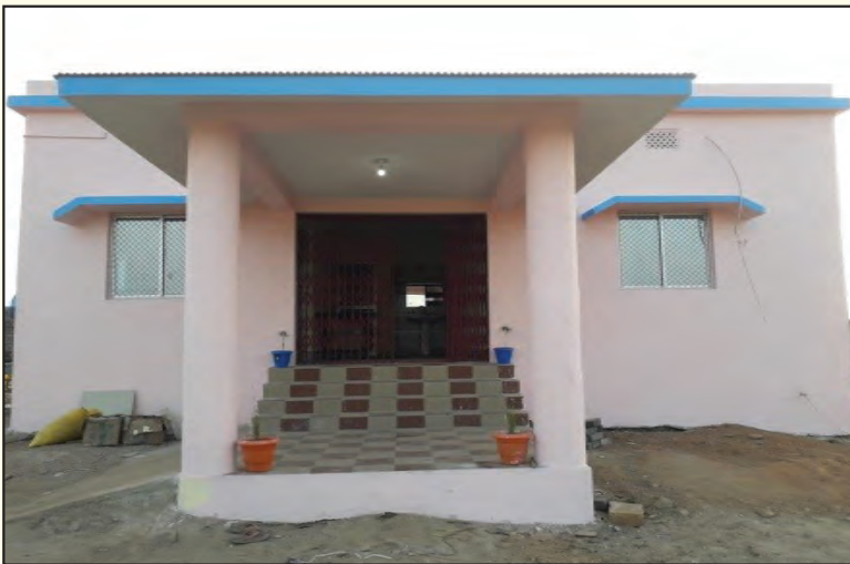
Office Building & Laboratory at WTP, Champua, Keonjhar District
