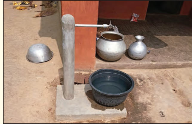
FHTC (Tap connection at Rairangpur)
