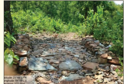
Loose Boulder Check Dam
