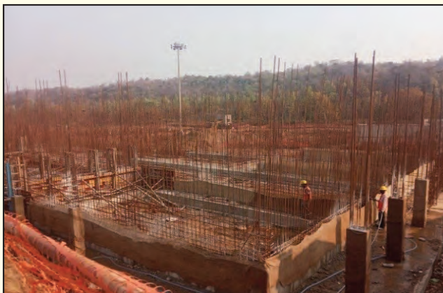
Construction work in WTP Site at Pallahara Block, Angul
