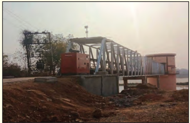
Intake Well, Mega PWS to Adaghat & 121 Villages, Sundargarh District
