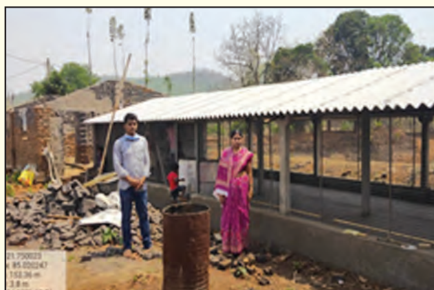
Construction of Poultry Shed, Sundargarh
