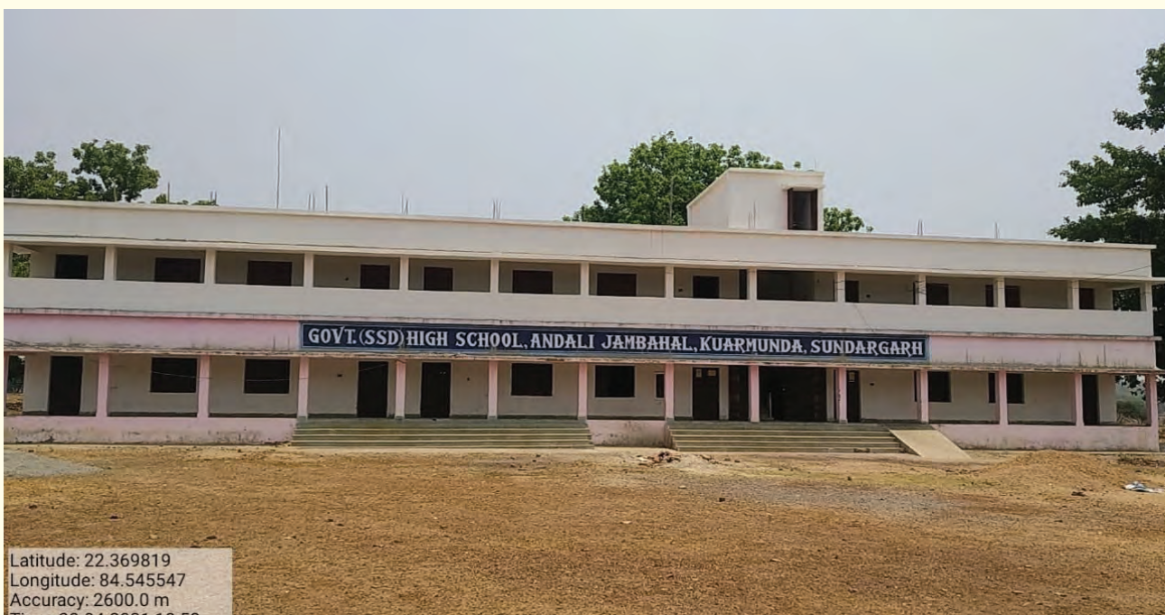
Construction of Library Room, ITDA Sundargarh
