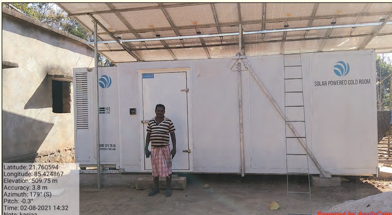
Installation of 5 MT Solar Cold Chamber, Madhyapur, Harichandanpur, Keonjhar
