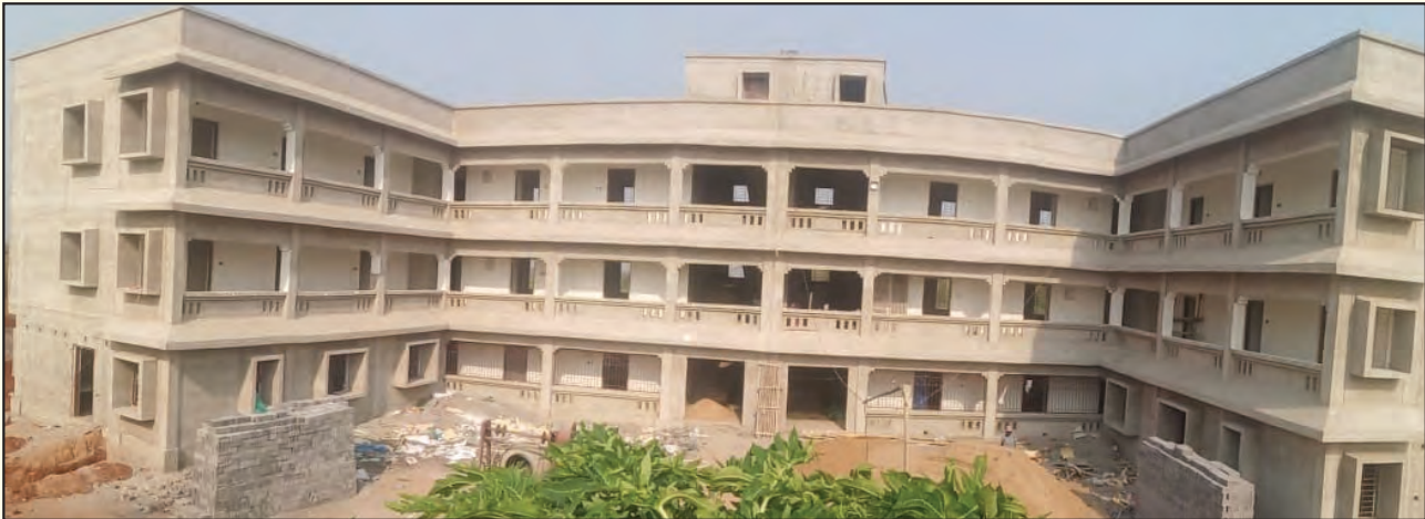
Construction of Hostel Building (Boys & Girls) at SDC-Bankisole, Baripada, Mayurbhanj
