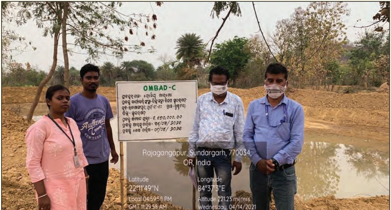
Excavation of new ponds for fish farming, Rairangpur, Sundargarh
