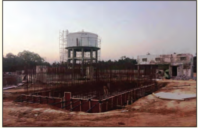
WTP Site Mega PWS At Rajgangpur, Sundargarh District
