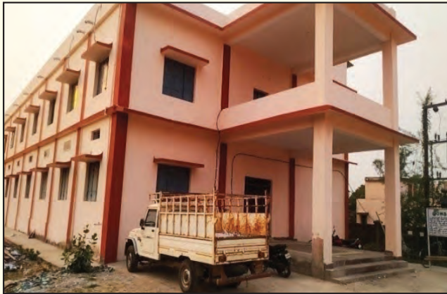
Construction of Drug Warehouse at DHH Sundargarh is completed.
