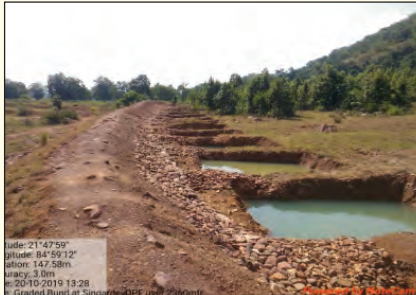
Earthen Graded Bund
