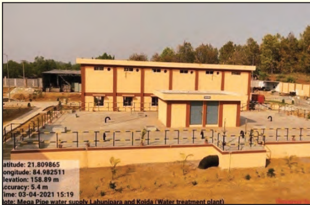
WTP Site Mega PWS to Adaghat & 121 Villages, Sundargarh District
