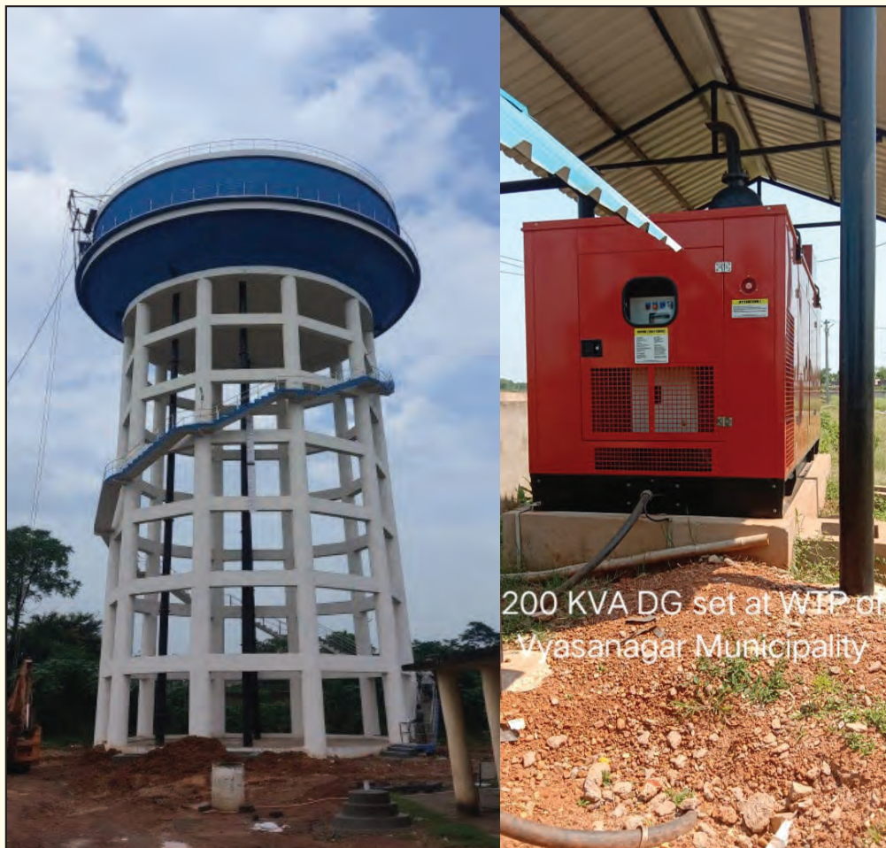
Completed Overhead Reservoir at Rourkela Township Area, Sundargarh District
